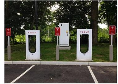
When both pairs of Tesla Supercharger station stalls (A and B) occupied, they share the available power of up to 150 kW. However, the depicted Superchargers are the older generation, only capable of delivering 105 kW per car.<sup>[14]</sup> Each Supercharger cabinet<sup>[15]</sup> with twelve charger modules<sup>[16][17][18][19]</sup> feeds two charging stalls (max 150 kW per car), so if two cars are charging at the same time their charging rate may be reduced.<sup>[20]</sup>
